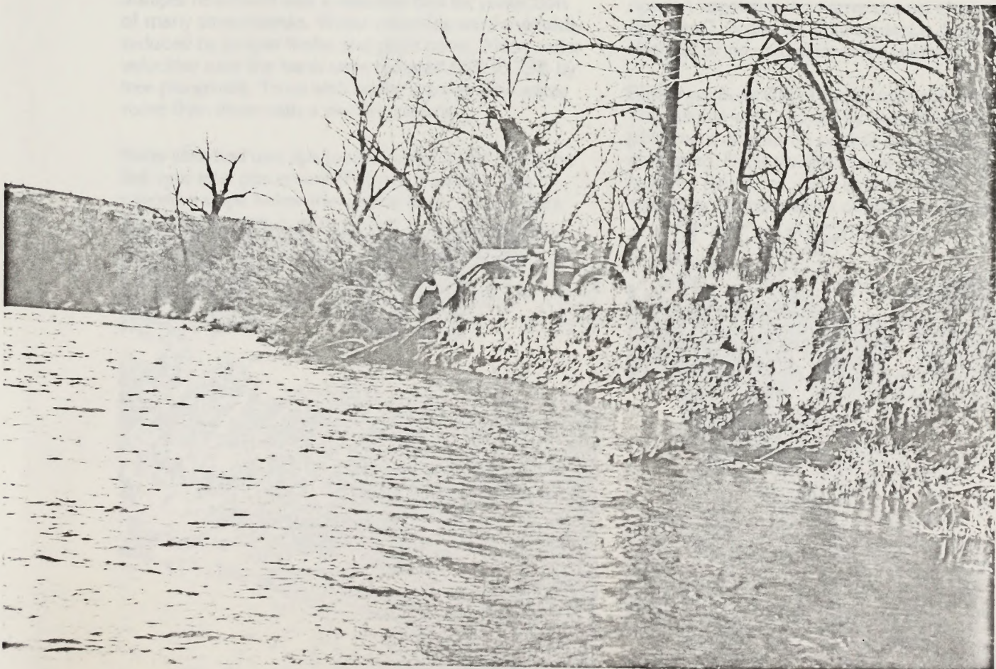
Figure 2 Tractor used in placing junipers on eroding bank.
